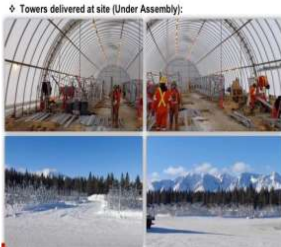
Figure 22: Tower assembly in gas heated tents and assembled structures at site
