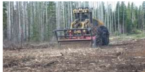
Figure 18: Tree cutting & cleaning in transmission line corridor
