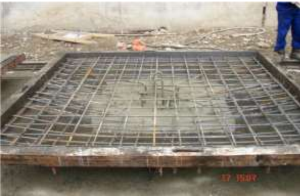
Figure 25: Reinforcement used in the base and chimney of foundation
