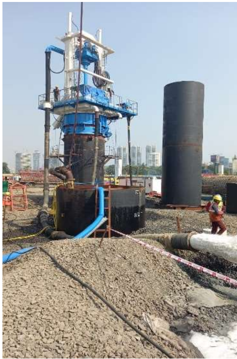
Figure: 2 A Reverse Circulation Drilling Rig in operation
