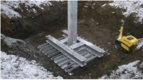
Figure 21: Steel grillage lowered in foundation pit.
