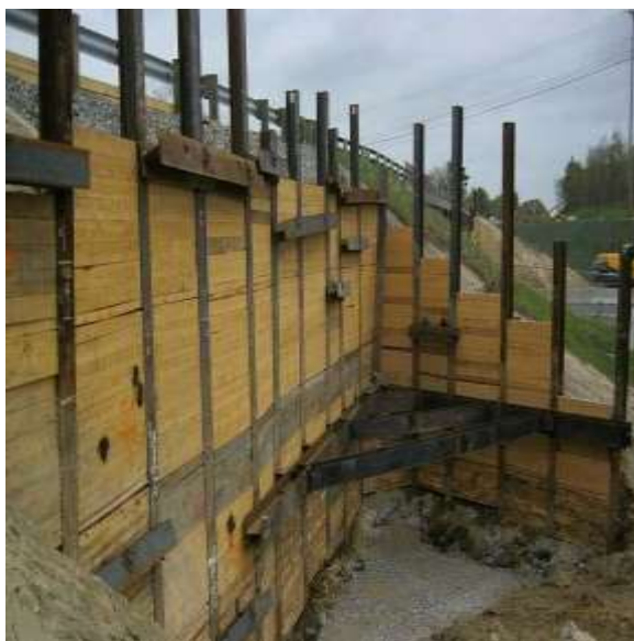
Figure 2 Importance of shoring in construction works
