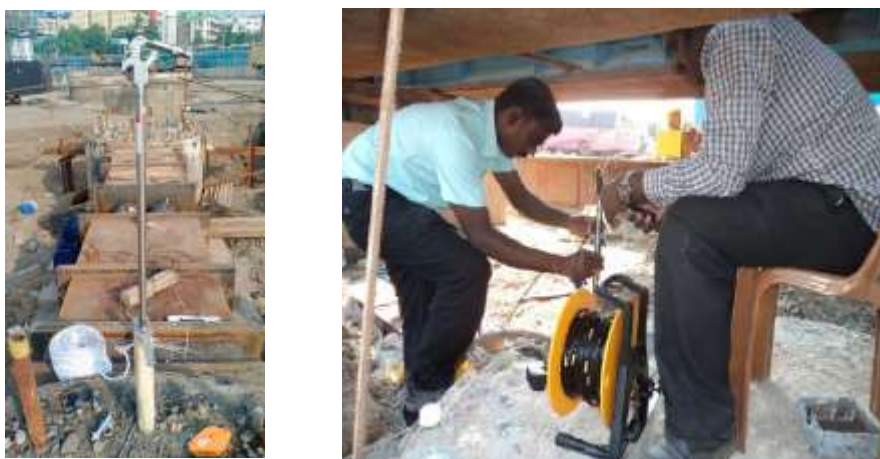
Figure: 9 In-place inclinometer and testing with torpedo type inclinometer on right
