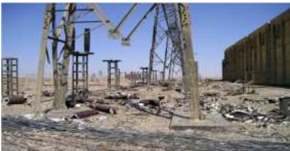
Figure 9: Fully damaged sub-station during the war
