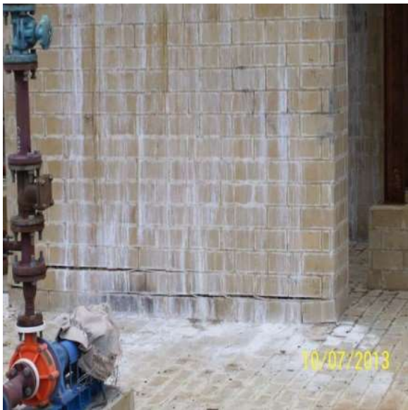
Figure 1A & 1B Settlement and crack development due to improper
