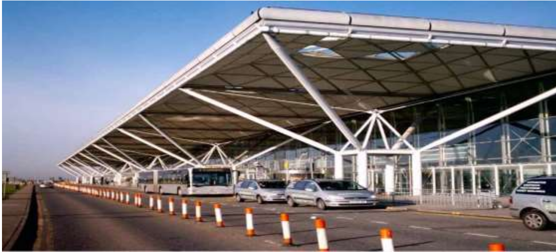
Figure 2: Stansted Airport displays the use of steel modules to provide long span and other design features that enhance its sustainability.
