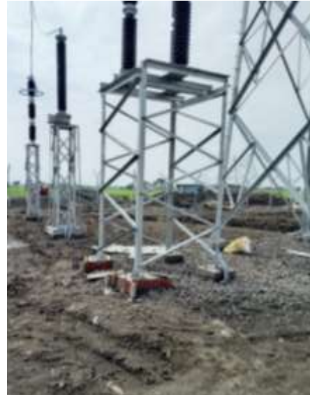
Image 1: Photographs of tilted/settled foundations
