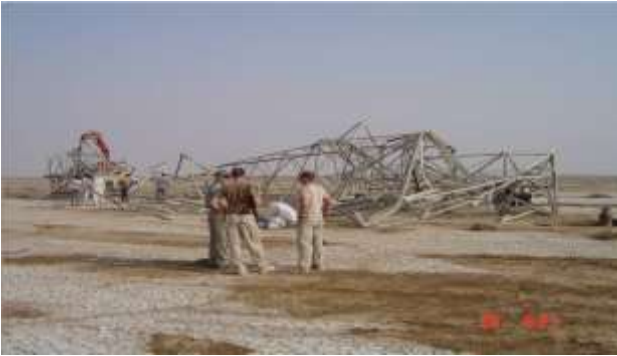
Figure 8: Inspection of damaged tower during an assessment study
