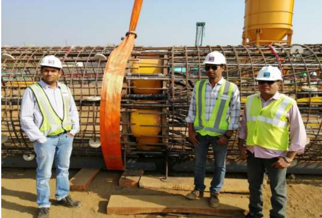
Figure: 4 Bi-Directional Assembly ready for lifting and lowering
