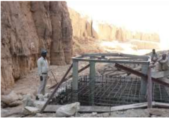
Figure 15: Block Foundation in progress along with Template
