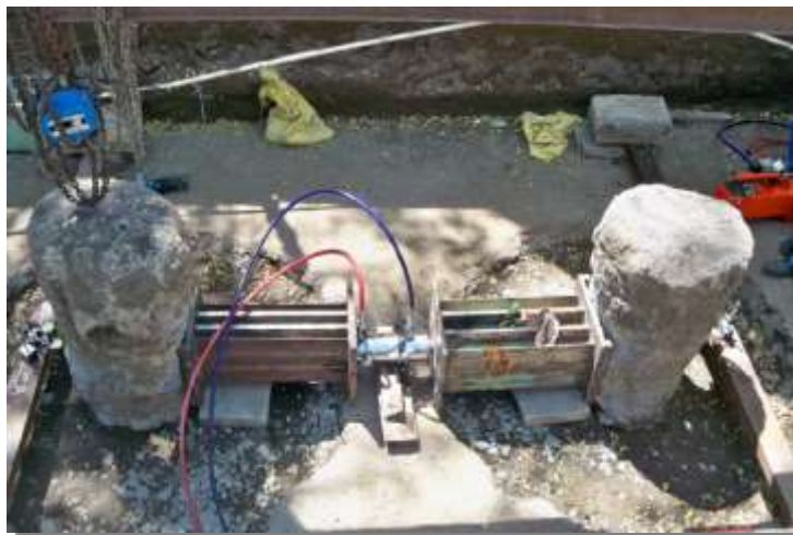
Figure: 8 Conventional Lateral Load Test in progress
