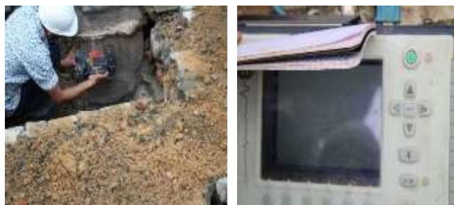
Figure-1 Testing of cover by a meter
