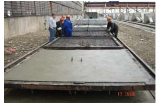
Figure 27: Mass production of precast foundations in plant
