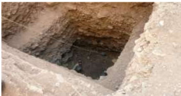
Figure 16: Deep excavated foundation
