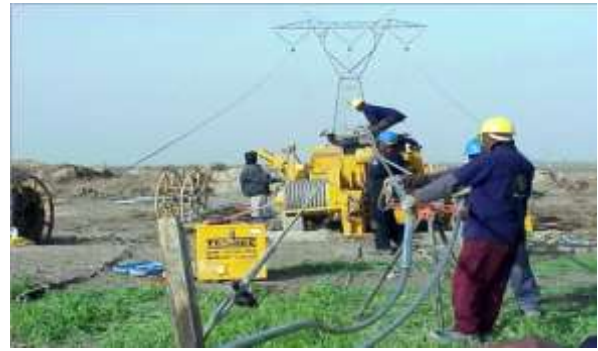
Figure 90: Final restoration work in progress
