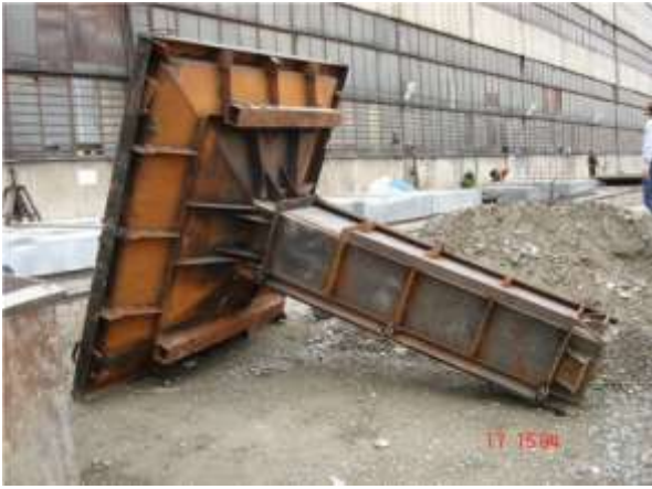
Figure 24: Form-Box for pre-cast foundation (base & chimney)
