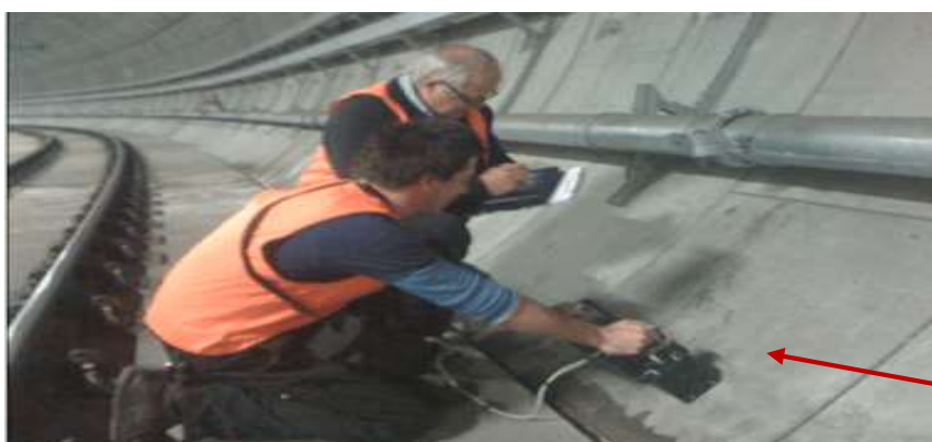
In Railway Tunnel
