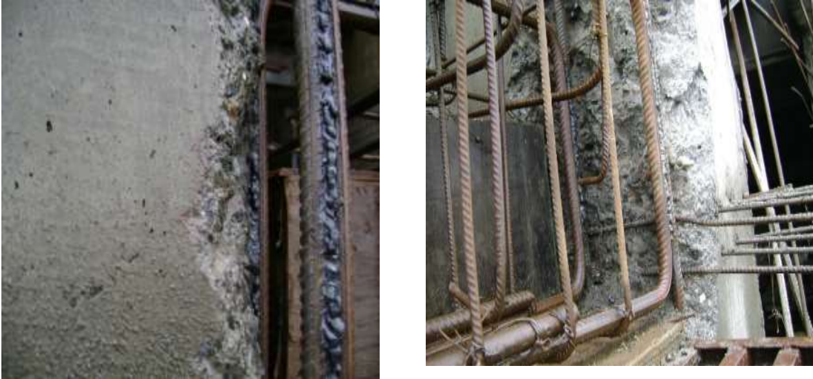
Figure 10 Rework due to error in civil drawing
