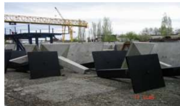
Figure 28: Final precast foundations are ready
