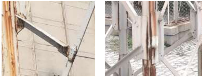
Figure -5 Joints at Column C9 bay IT feeder 2
