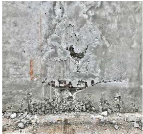
Figure 4 A & B Slurry Leakage & Segregation of Concrete
