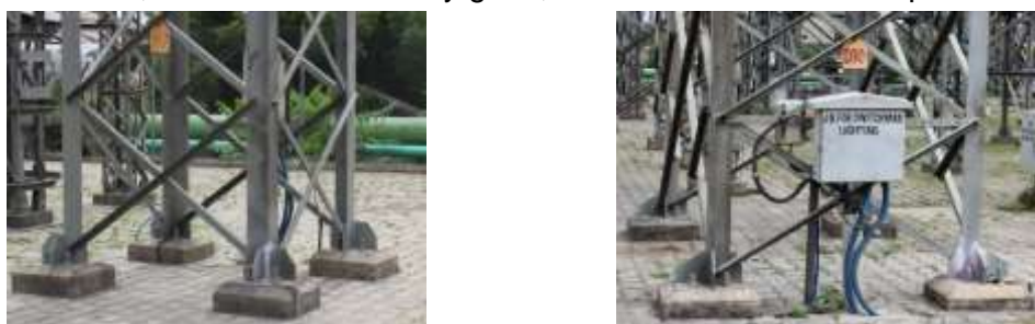
Figure 8 foundations in 132kV (Airport)
