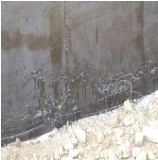
Figure 7 Honey Combing in Concrete
