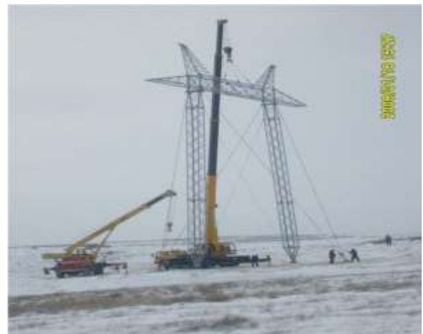
Figure 23: 500kV Single Circuit double mast auved tower under construction
