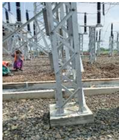
Image 2: Photographs of tilted/settled foundations
