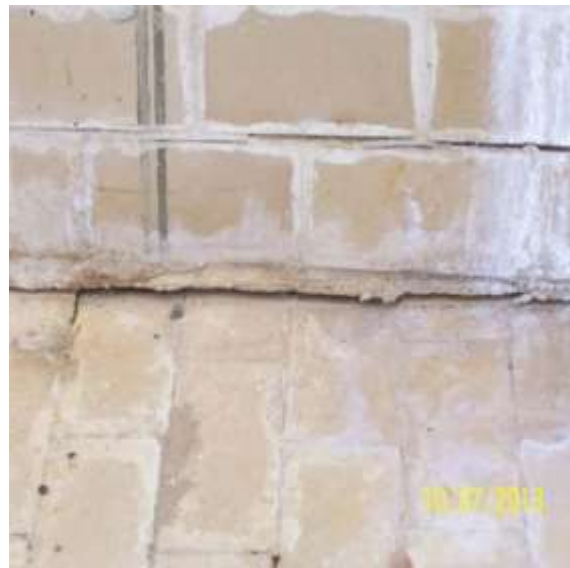
Figure 1A & 1B Settlement and crack development due to improper
