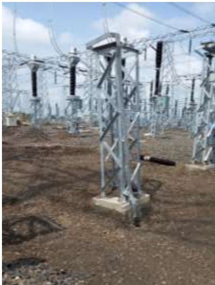
Image 1: Photographs of tilted/settled foundations
