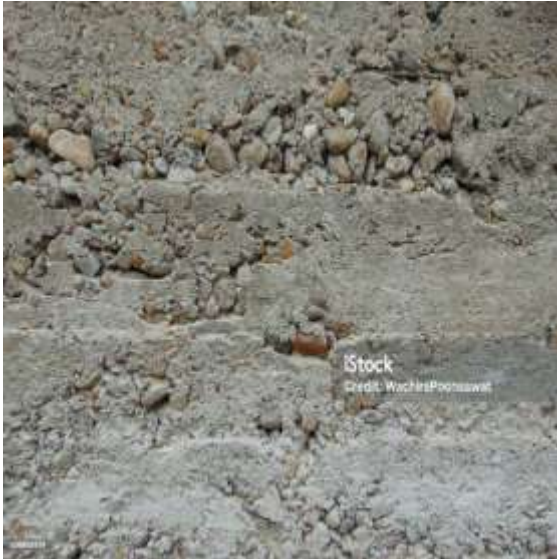
Figure 4 A & B Slurry Leakage & Segregation of Concrete
